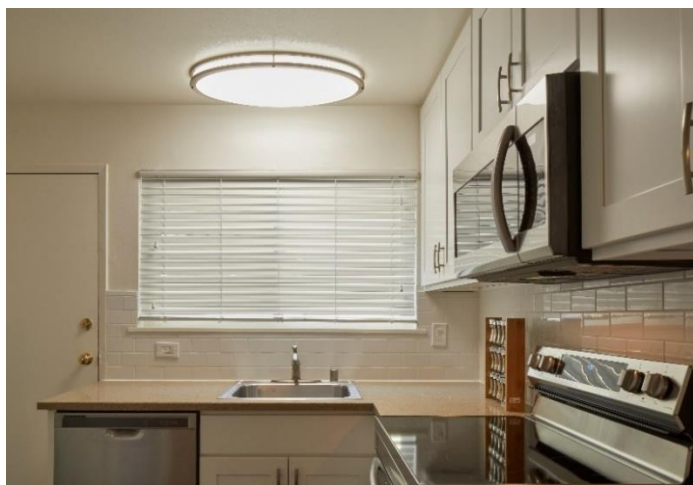
A renovated kitchen with LED lighting, low flow water fixture, and an induction cooktop
